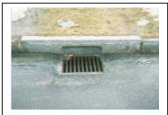
Drainage inlets typically lead to pipes that become stormwater point source discharges
