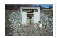
Outlet structure for detaining a range of flows
