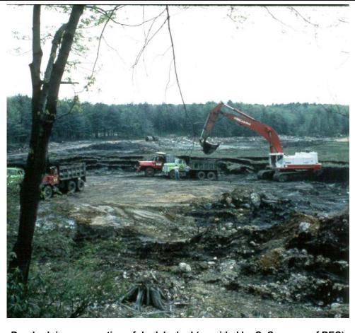
Dry dredging: excavation of dry lake bed (provided by C. Carranza of BEC)
