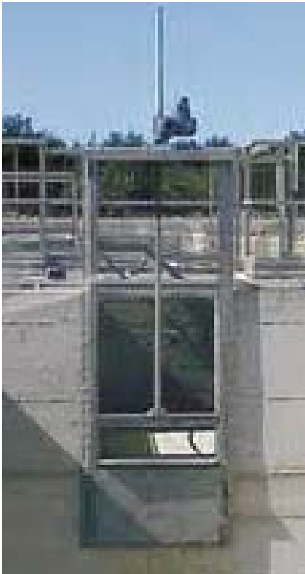
Figure 8 Weir Gate With Electric Actuator
