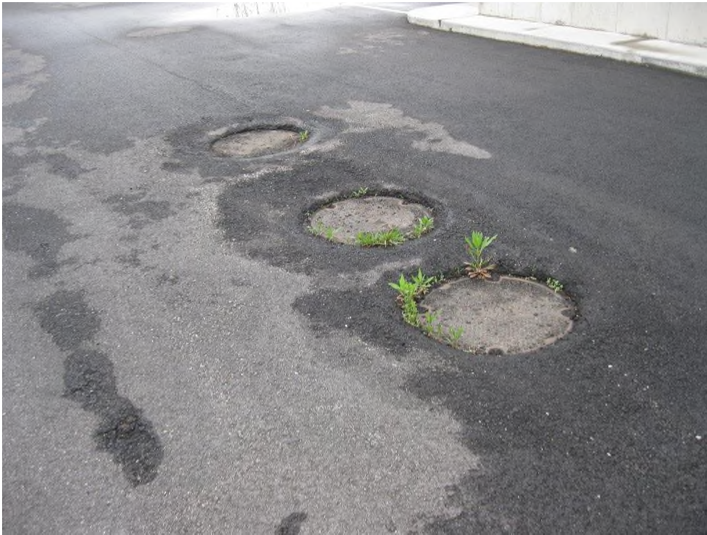
Recessed septic tank covers.
