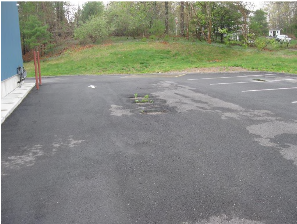
Recessed septic tank covers.
