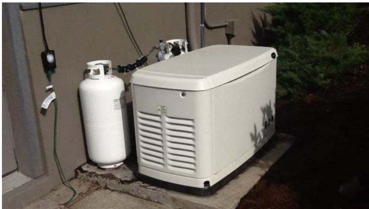
Figure 6 Propane-Powered Generator
