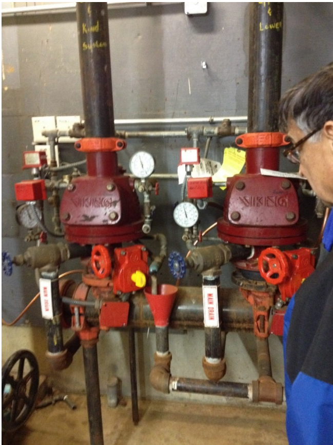
Photo 5: Dry pipe valves and accessories
