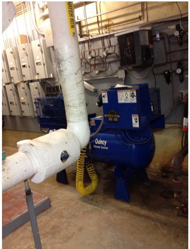
Photo 4: Temporary Air Compressor for Dry Pipe System
