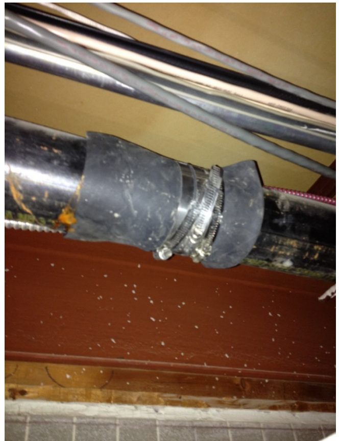
Photo 8: Temporary patch for leaky pipe
