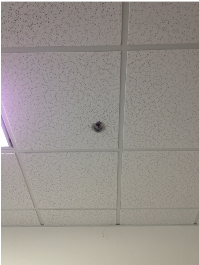
Photo 7: Pendant sprinkler head
