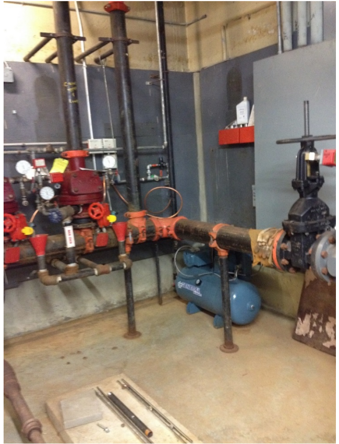
Photo 2: Dry Pipe Risers
