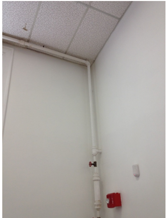
Photo 6: Sprinkler Drain
