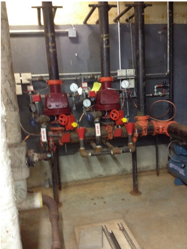
Photo 3: Dry Pipe Risers
