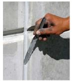
3. The final main feature of the backer rod is that is promotes an hour glass shape. This maximizes the bond area but keeps the depth of sealant consistent in the middle allowing for movement.
