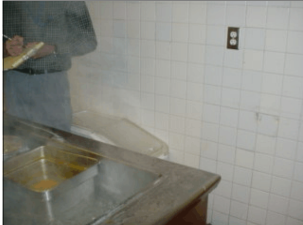
Figure 3: Outlet near a sink without necessary GFCI protection.
