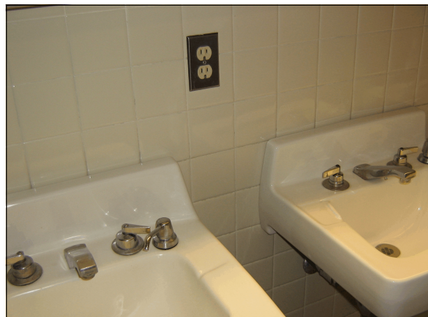
Figure 2: Outlet in a bathroom without necessary GFCI protection.
